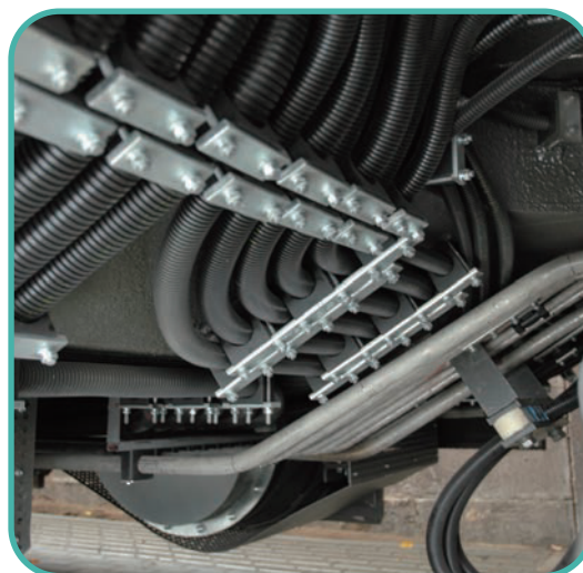
Under carriage installation 车下安装
